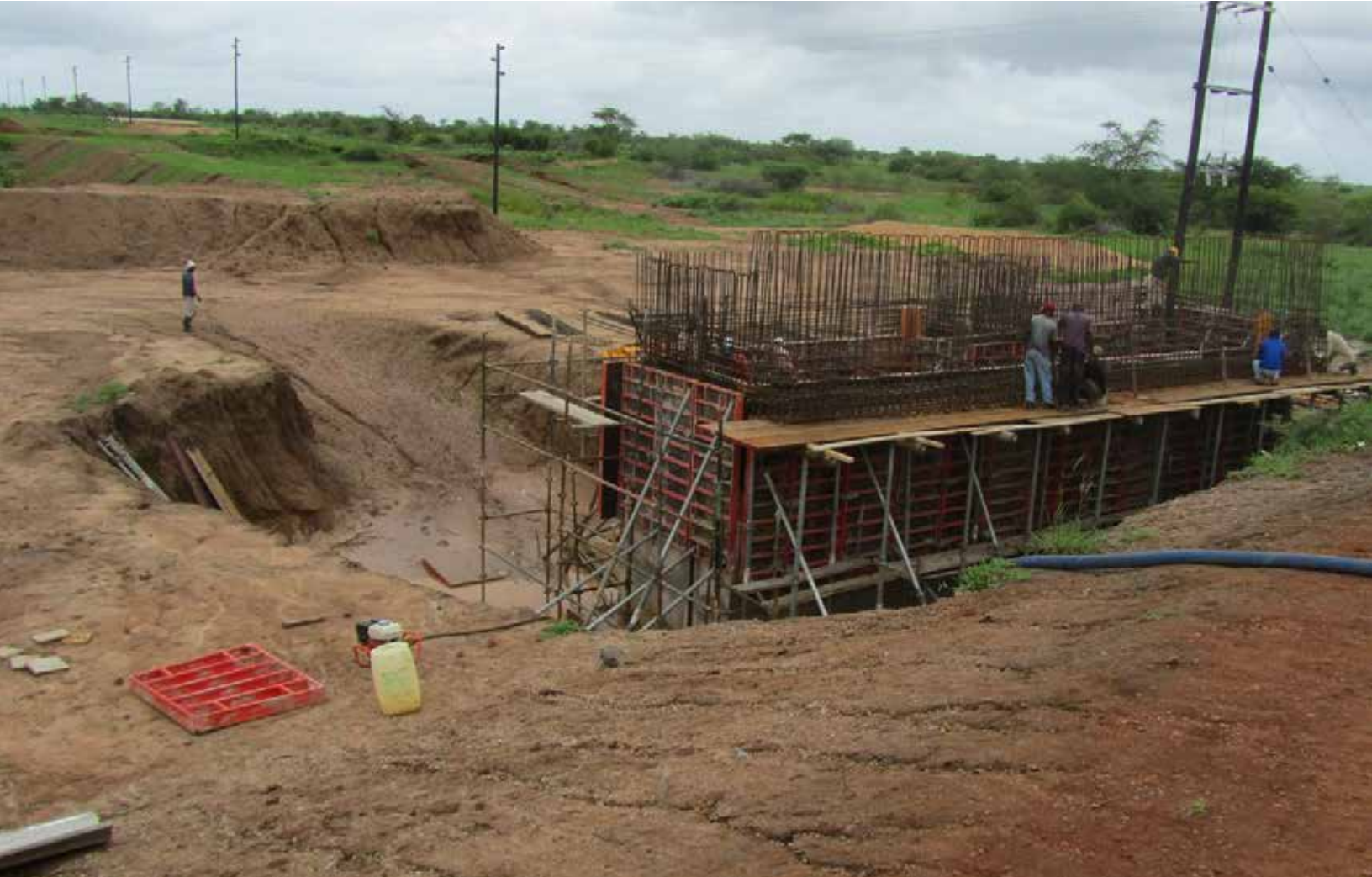
Putting in the pump to irrigate fields, Emvest Limpopo in Matuba
